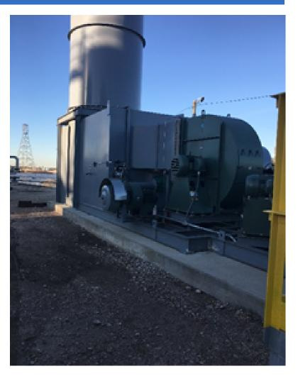
The VCU for this project is heated by an independent burner package in a vertical refractory-lined steel chamber. A small blower was provided to direct fresh air to the burner assembly for purging the system prior to ignition and to cool the burner assembly during operation.
